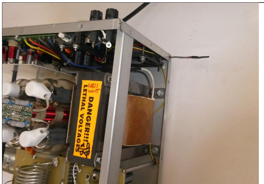
Figure 8 pull wire once through
